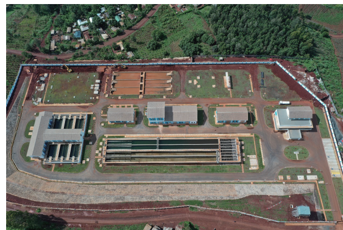
A panorama view of the water plant project ▶
