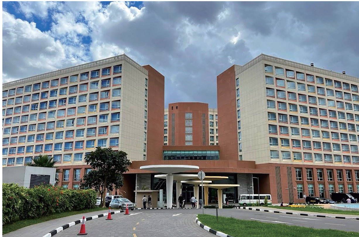
▲ Ethiopian Skylight Hotel Phase II
