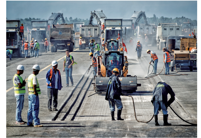
▲ Site of Bandaranaike Airport runway project, Sri Lanka
