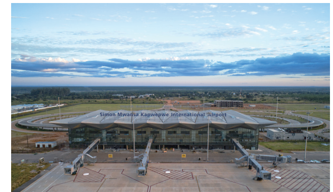
Ndola International Airport ▶
