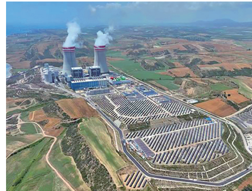
▲ The aerial view of the Hunutlu coal-fired power plant
